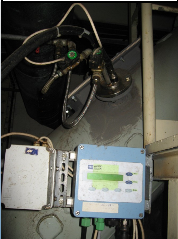
HK2 pin antennas with cleaning function Sugar
